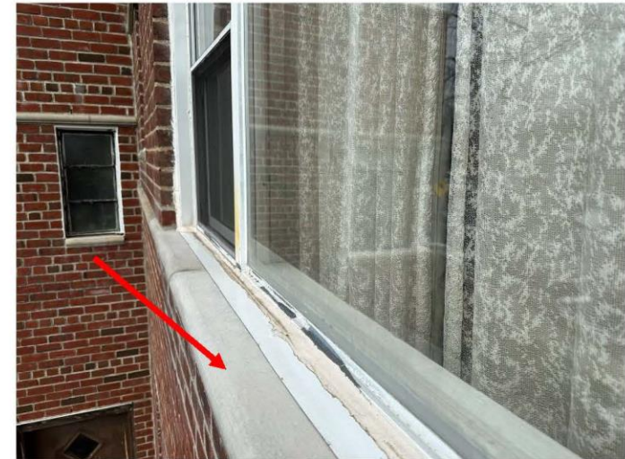
Photo-4: Building No. 1: 196-15 Dunton Avenue. Close-up view of properly installed windowsill.
